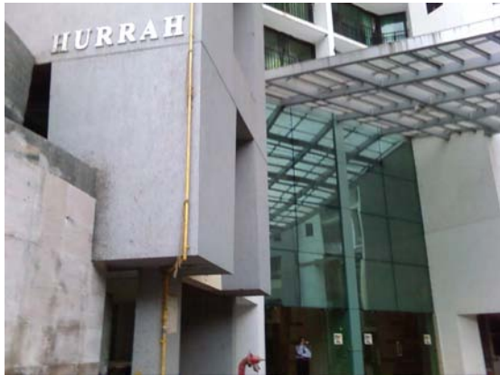
Figure 2: Facade of the HURRAH residential tower currently and enthusiastically under construction.
